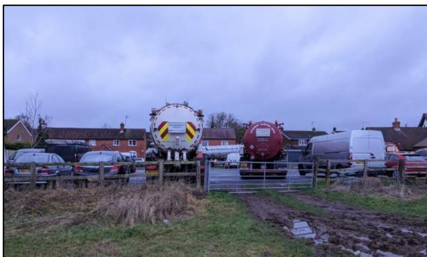
Tankers in The Plough car park used for taking away sewage from pumping station.
