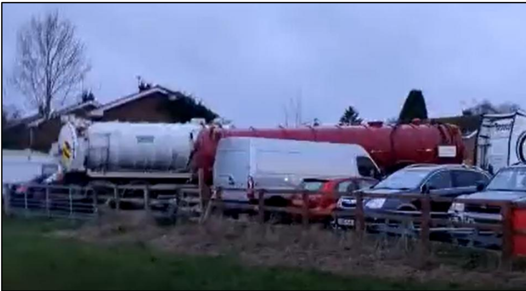
Tankers in The Plough car park used for taking away sewage from pumping station.
